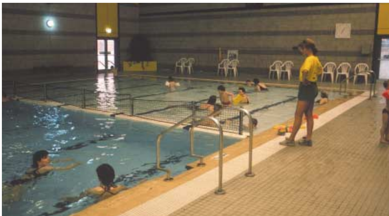
The introduction of a moveable floor and bulkhead eliminates the need for a separate teaching pool and should eliminate the need for a separate toddlers pool, helping to reduce energy and staffing costs.
