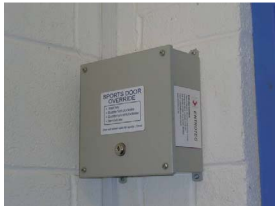
Image 6: Manual over-ride box (above) Image 7: Push-bar exit
