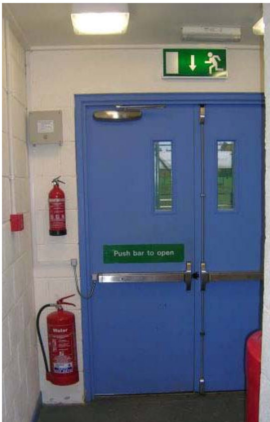
Image 6: Manual over-ride box (above) Image 7: Push-bar exit
