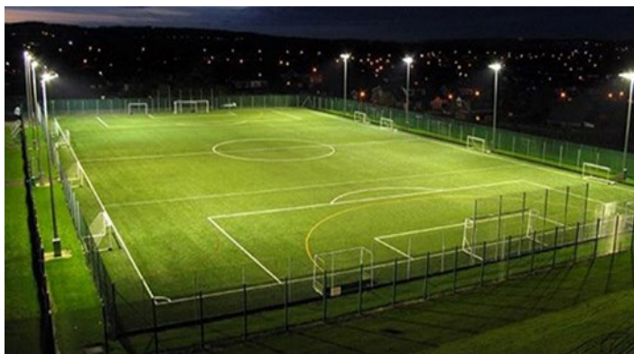
3G pitch at Craigie Sports Hub, Dundee – 8 floodlighting masts allowing the pitch to be split into thirds.
